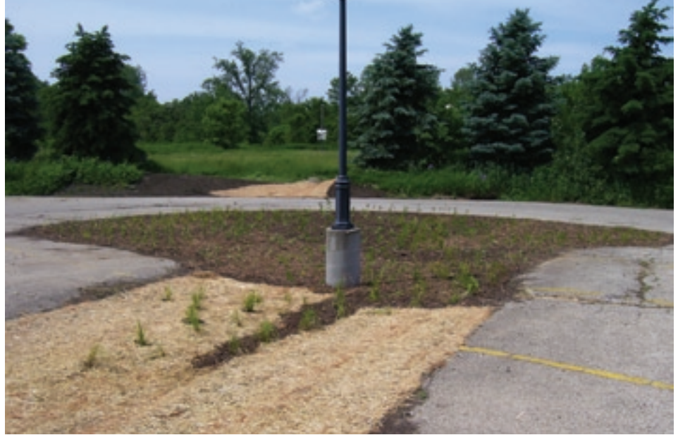
Bioretention areas are among practices recommended by the Elkhart River Alliance in its efforts to restore health to the Elkhart River Watershed. The Elkhart County Soil and Water Conservation District is joined by other partners in the effort.
