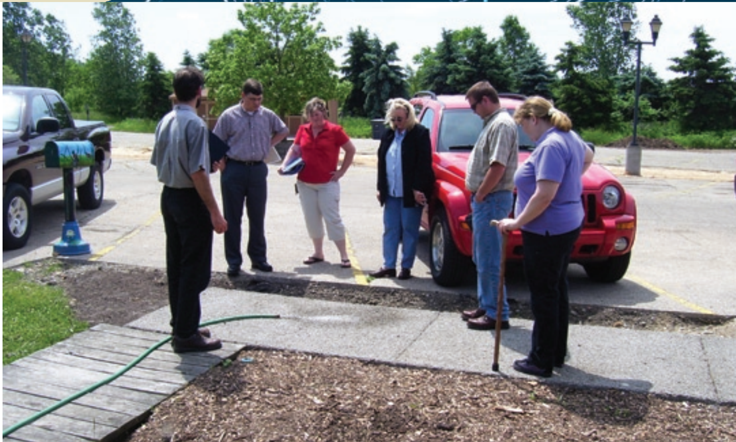
Pervious pavement at the city of Elkhart Environmental Center increases on-site storm water infiltration. It is among many practices recommended by the Elkhart River Alliance.
